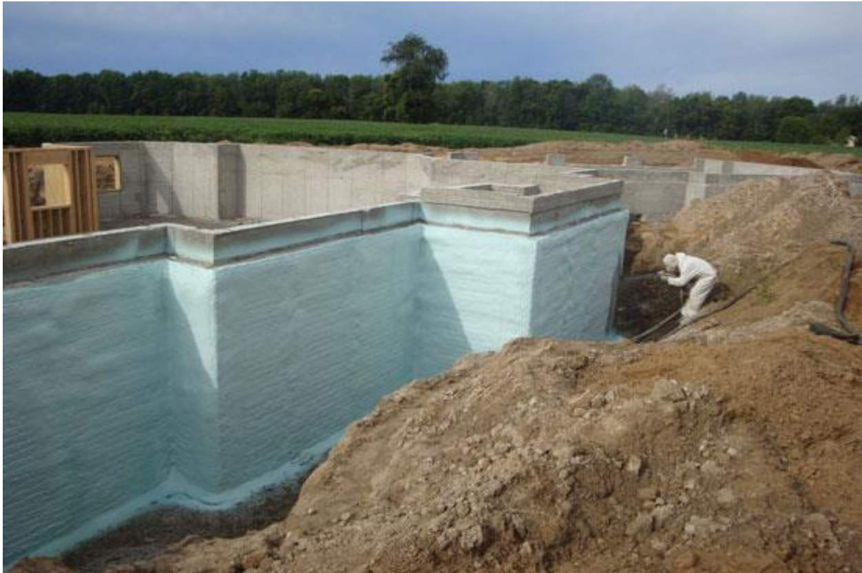
Figure 3 – Exterior below-grade wall installation (photo)
