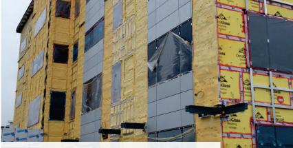
**Profoam** Proudly Introduces **HYBRID Pro 1.0**, The First Vapor Permeable Exterior Polyurethane Foam Used As A Thermally Insulated Sheathing Membrane.
