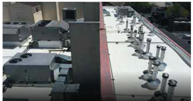
SPF provides self-flashing around all deck-mounted equipment and penetrations for this industrial manufacturing facility.
