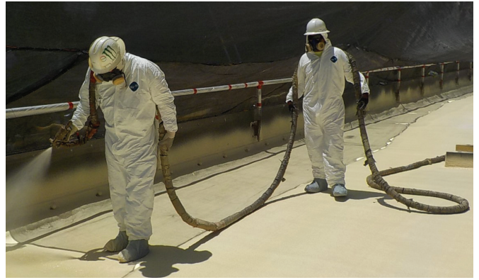
Application of ProZone on a low-slope roof.
