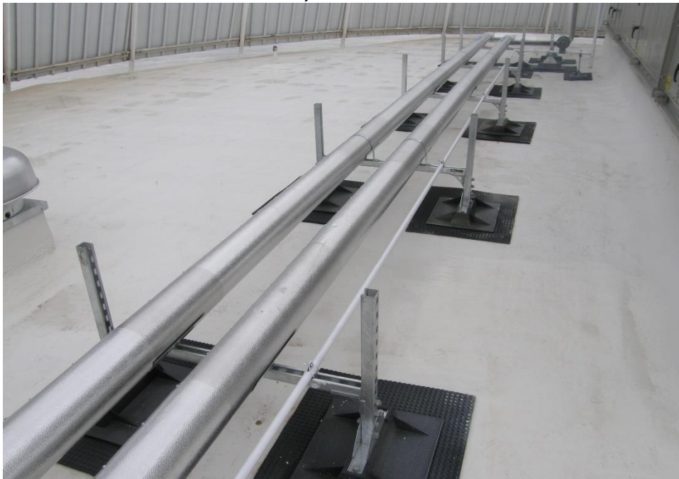
Figure R7-4: Piping system properly installed and elevated on support pads above the roof Courtesy Bruce Schenke
