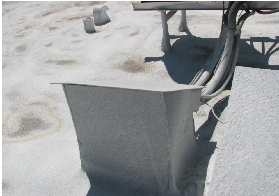
Figure R7-5: Power cables properly installed from roof penetration housing to load Courtesy Mason Knowles Consulting
