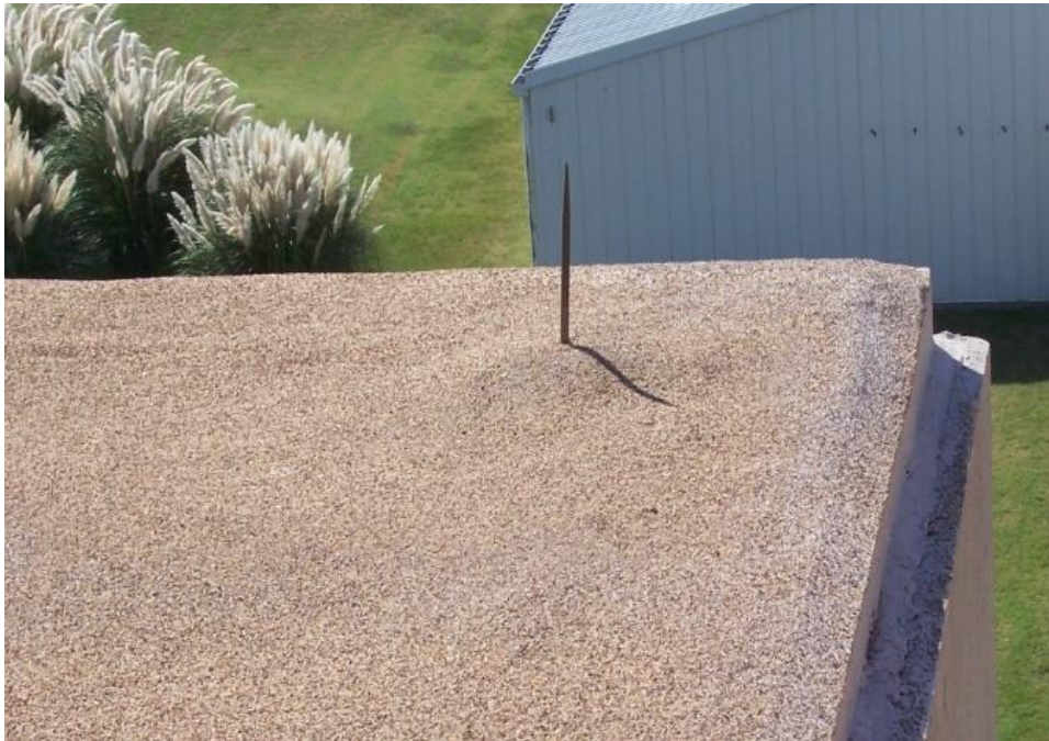
Figure R7-2: Lightning arrest cables improperly covered by a SPF roofing system
