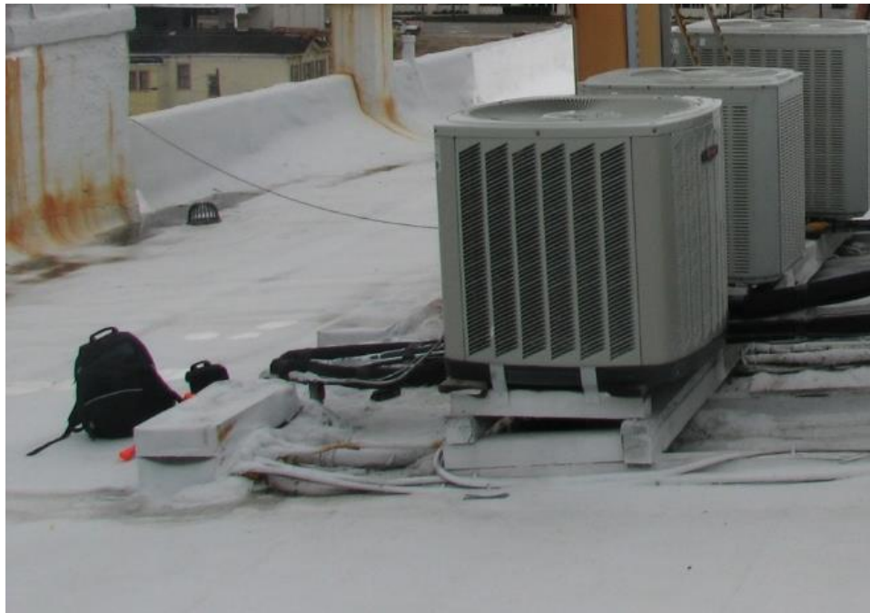
Figure R7-1: Power cables and piping improperly covered by a SPF roofing system Courtesy Mason Knowles Consulting:
