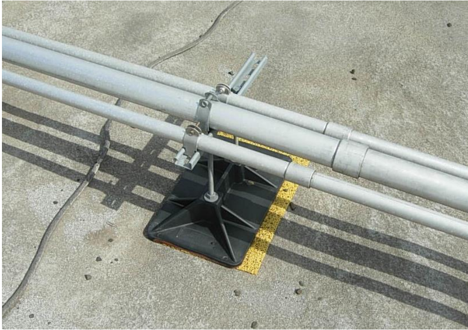
Figure R7-3: Power cables properly installed in conduit elevated on support pads above roof Courtesy Bruce Schenke
