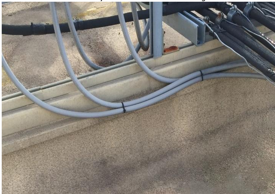
Figure R7-6: Wiring properly supported above roof on top of curb Courtesy Mason Knowles Consulting
