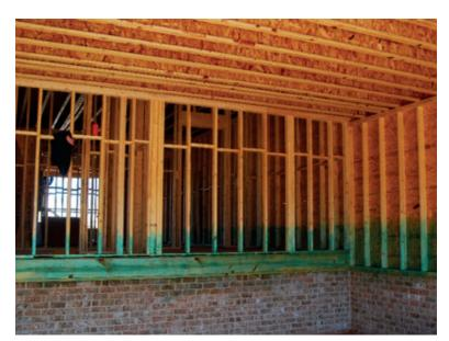
FIGURE 6. Borate treatment of select structural wood components
