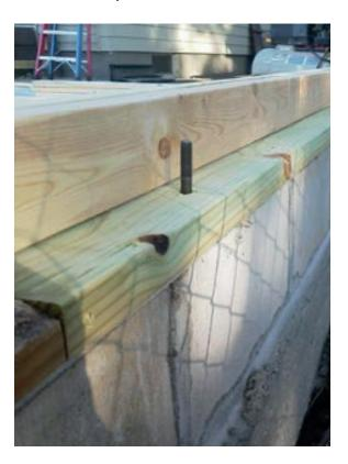
FIGURE 9. Termite resistant preservative treated wood near the foundation
