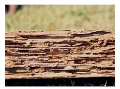
FIGURE 5. Evidence of structural termite damage
