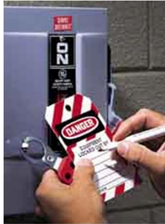
FIGURE 3 - Deactivate and mark HVAC system at electrical panel (use LOTO procedure and indicate date, time and name of person applying the tag).
