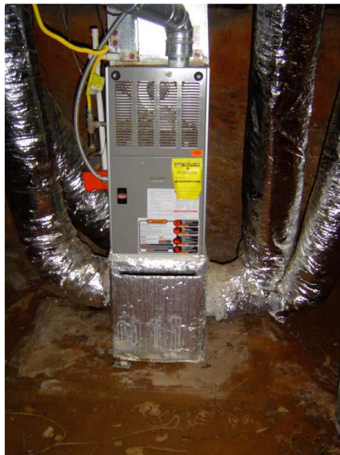
Figure I3-5: Draft fan-assisted HVAC system in a crawl space.
