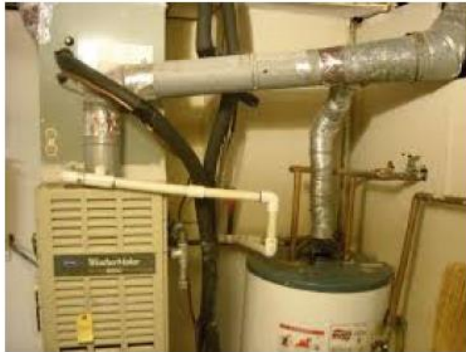
Figure I3-2: Typical open-combustion furnace co-vented with open-combustion water heater. (Requires fresh air source.)
