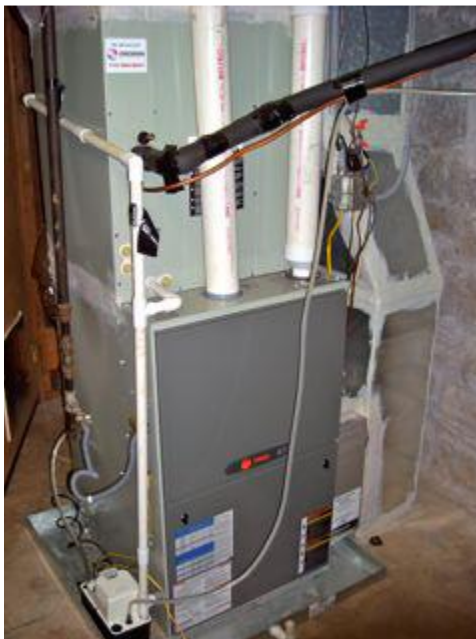
Figure I3-6: Typical sealed-combustion HVAC system. Air supply and exhaust is through the PVC piping. (No special requirements when air sealing building.)
