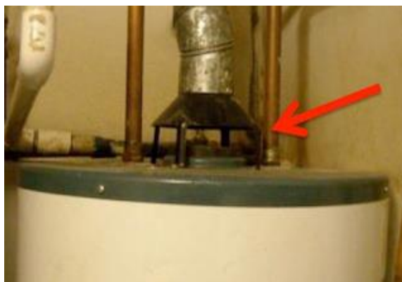
Figure I3-1: Typical open-combustion water heater. Arrow indicates the entrance to the exhaust flue.
