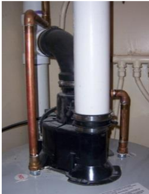
Figure I3-4: Powered vent on a water heater.
