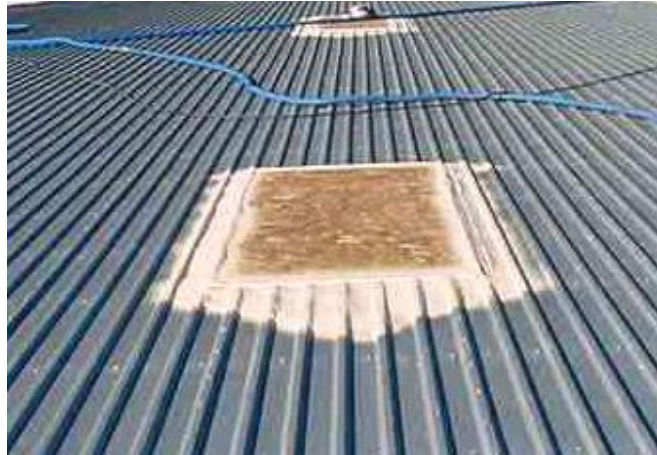
Figure R6-3: Completely remove existing skylights and reinforce openings before application of SPF roofing.
