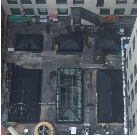
Figure R6-1: Existing skylights on older buildings may be covered with SPF roofing for insulation and air sealing without removal
