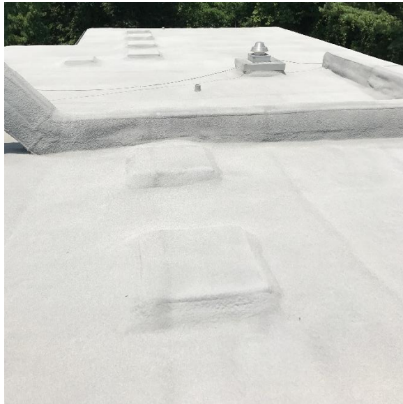
Figure R6-2: Reinforce existing skylights before application of SPF roofing. (The skylights are reinforced with dimensional lumber - not shown)
