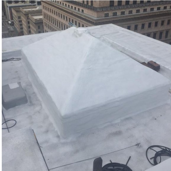
Figure R6-1: Existing skylights on older buildings may be covered with SPF roofing for insulation and air sealing without removal
