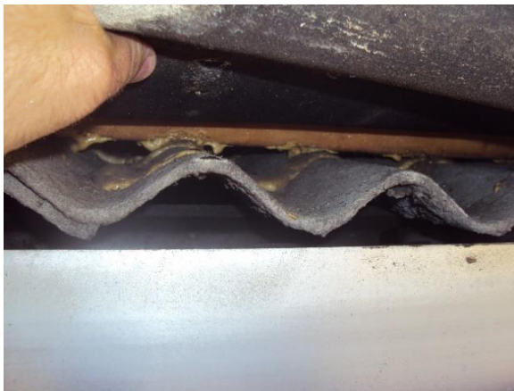
Figure 3 - Check Overall Condition of Transite, Including Fasteners
