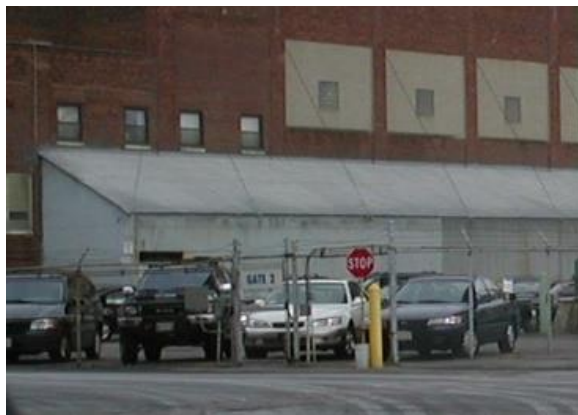
Figure 1- Example of a Sloped Transite Roof at a Manufacturing Facility
