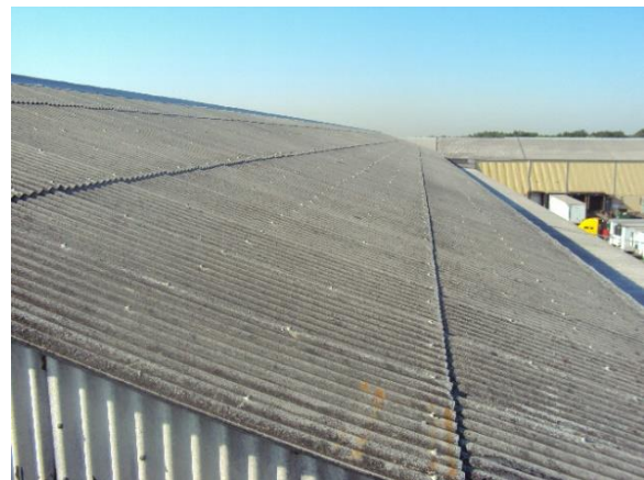
Figure 2 - View of Transite Roof Panels on a Sloped Roof
