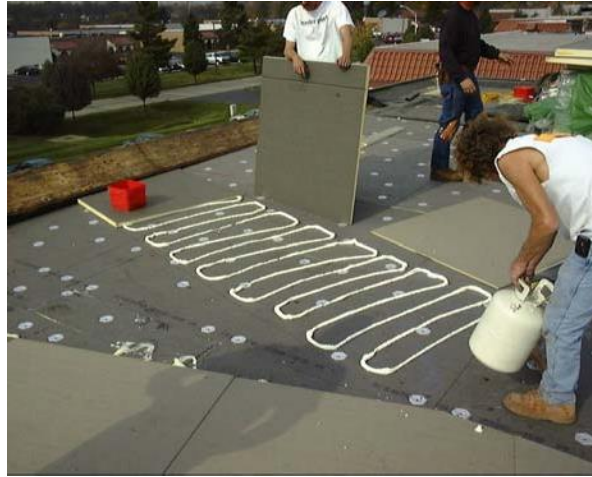
FIGURE 4: SPF ADHESIVE RIBBON APPLICATION
