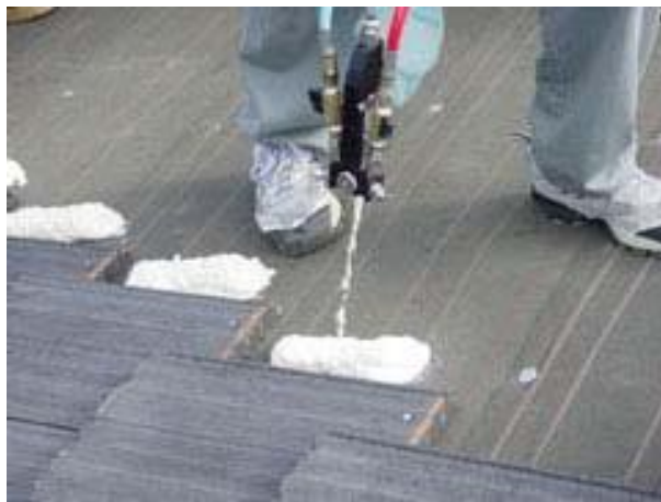
FIGURE 5: SPF ADHESIVE PATTY APPLICATION
