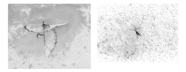
Coating damage can appear as gouges, cracks, and punctures. Hail-induced coating cracks often form patterns shaped like "crow's feet" or semicircles.
