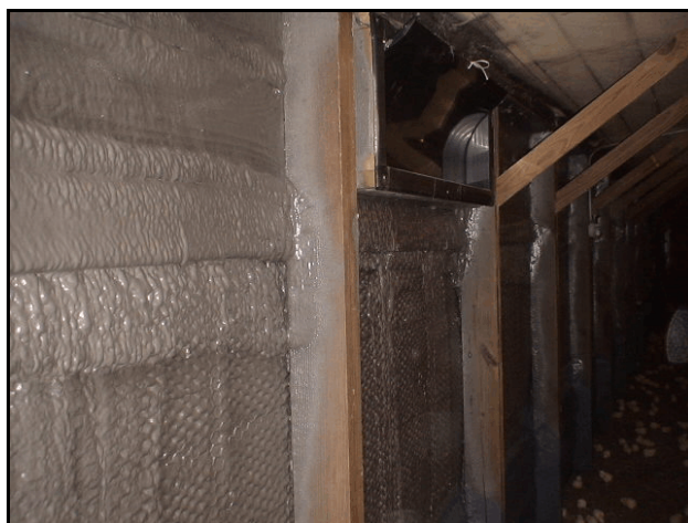
Figure 4. Side wall after polyurethane insulation was applied.
