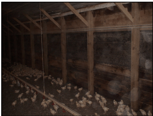
Figure 3. Side wall before polyurethane insulation was applied.
